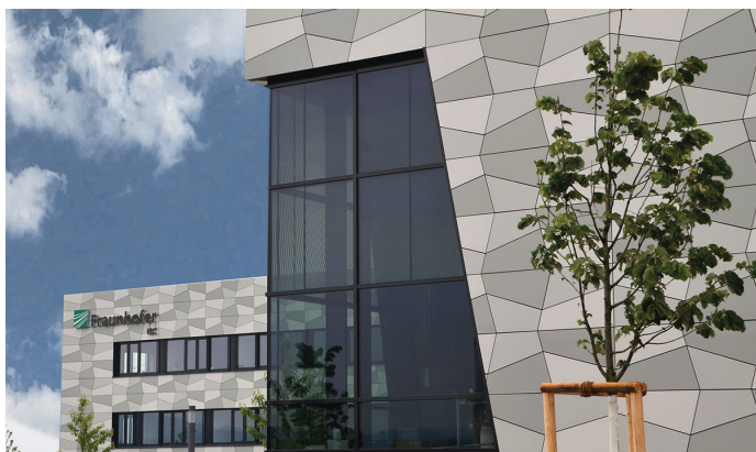
Fraunhofer-Center for High Temperature Materials and Design HTL in Bayreuth, Germany (Copyright: HTL)
